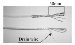
Strip approximately 50mm from the cable jacket, fold back the foil or braid shield, and separate the wire into 4 pair each.
